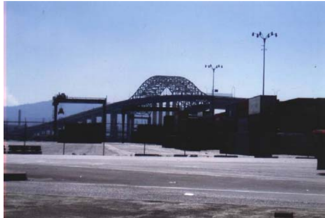
Terrorists use various types of weapons to carry out their objectives of fear, destruction and death. Some believe terrorists could target bridges to disrupt the flow of people and the economy.
