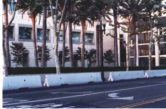
Concrete barriers in front of the Ronald Reagan Federal Courthouse in Orange County, Calif. are used as a precaution against criminal acts by terrorists.
